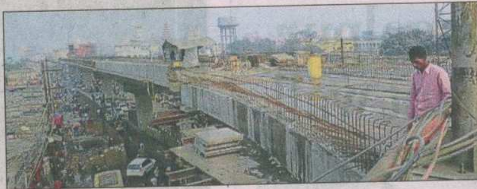
■ The under-construction Patna Junction flyover.
