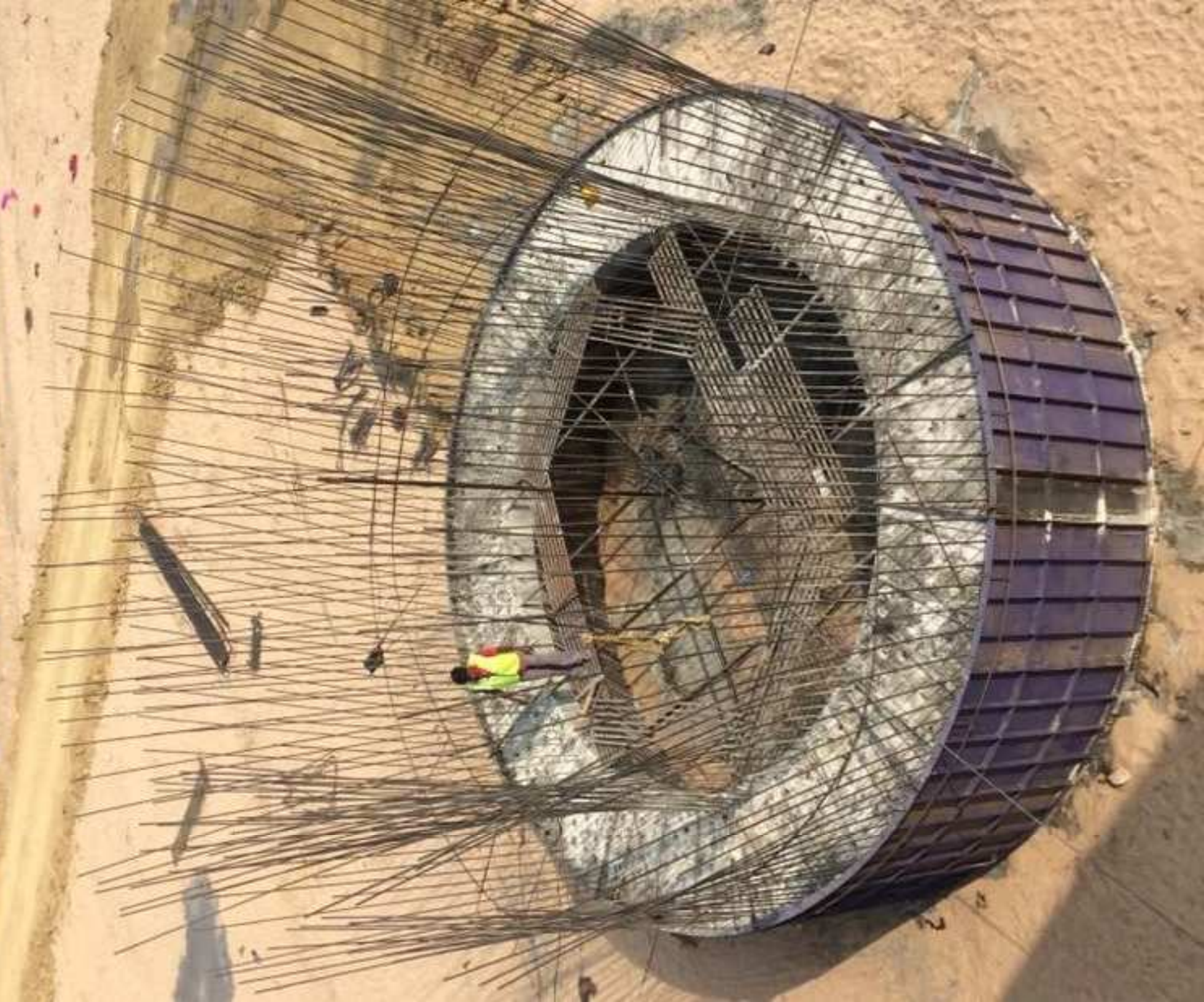
Well sinking at Falgu River Ch. 5th of NH-82
